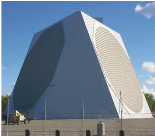
PAWS (US missile warning system from 1980): 2677 dipole elements
