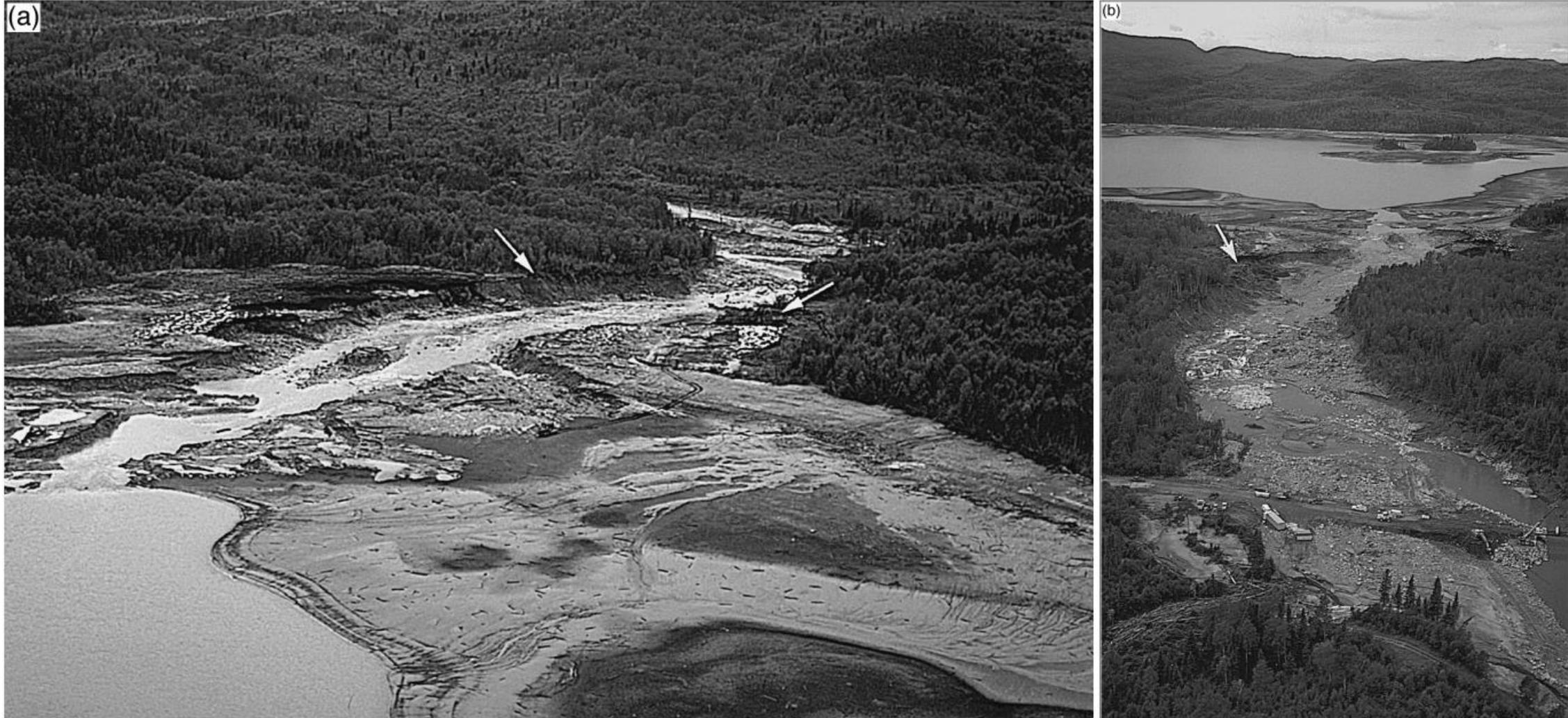
The new outlet at the Lake Ha! Ha! reservoir that was eroded through the Cut-away dyke, (a) looking downstream and (b) looking upstream. Source: Brooks & Lawrence (1999)
