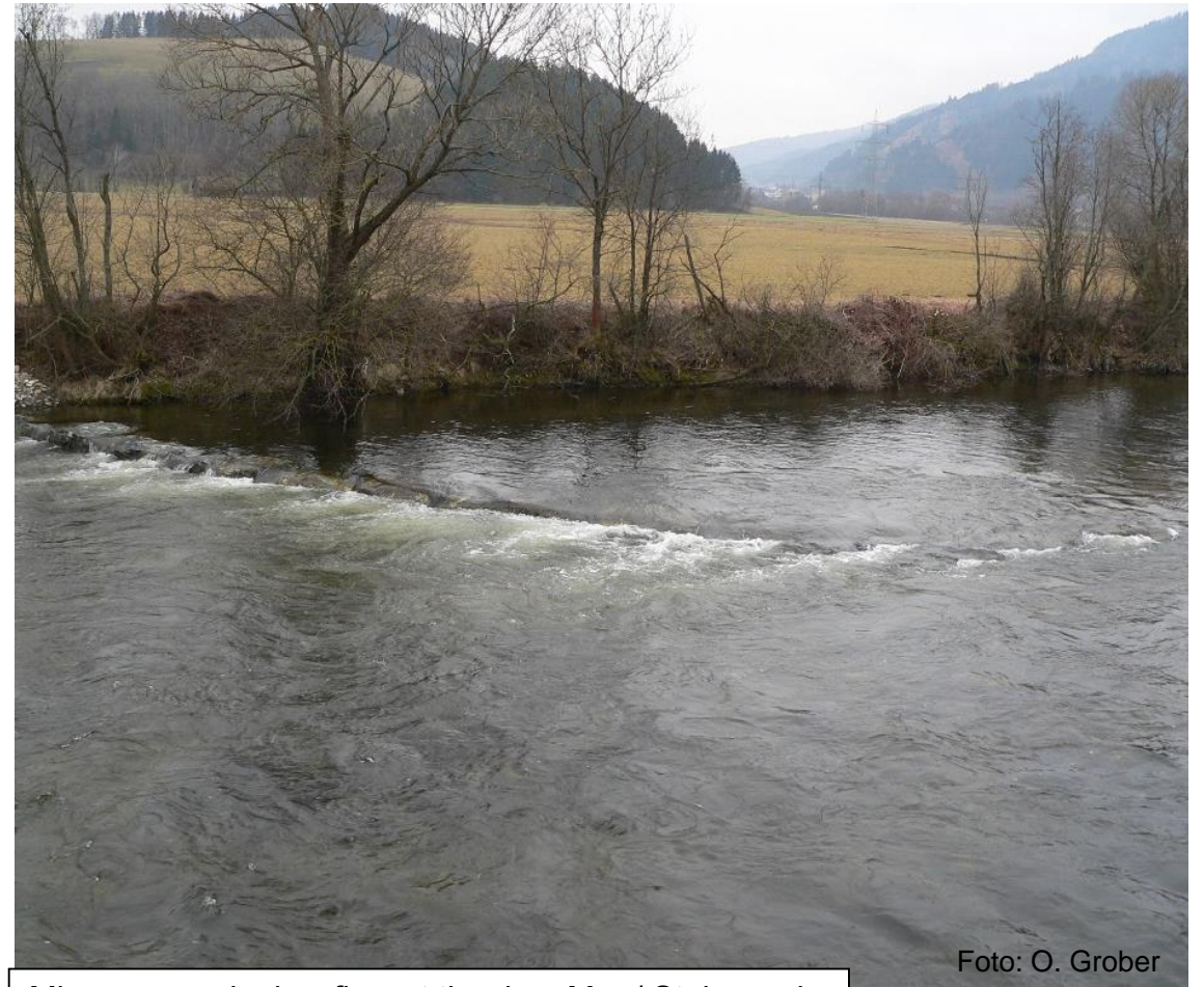
Micro groyne by low flow at the river Mur / Steiermark
