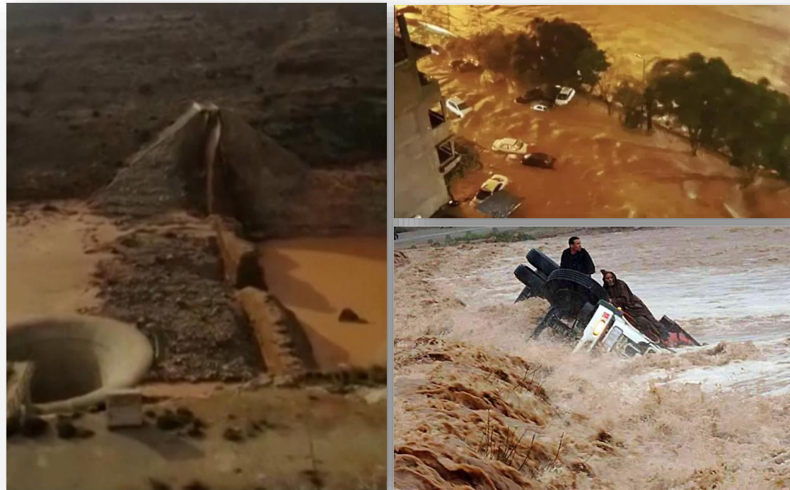
Derna Dams failure (Libya), September 2023
