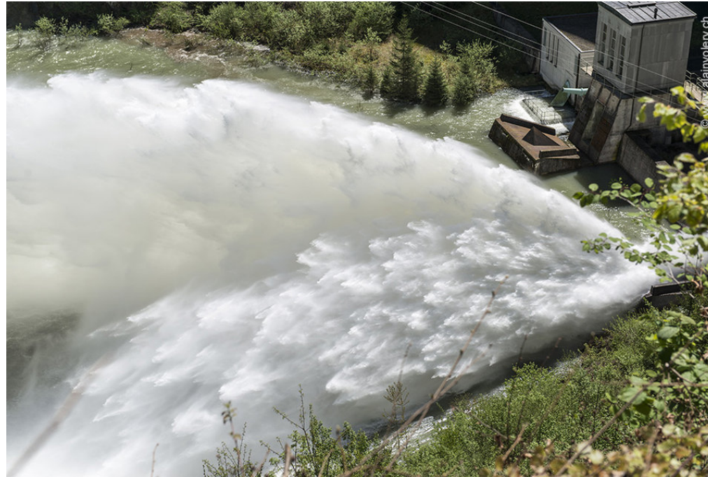
Water spill at the dam of Rossens. May 6, 2015 Source: www.lematin.ch
