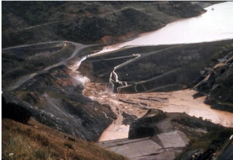
Initial surface erosion and deepening
