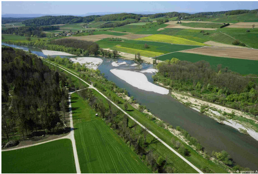
Figure 6.3 River widening at the River Thur near Altikon (ZH) in 2014, source: C. Herrmann, BHAtteam Ingenieure AG, Frauenfeld
