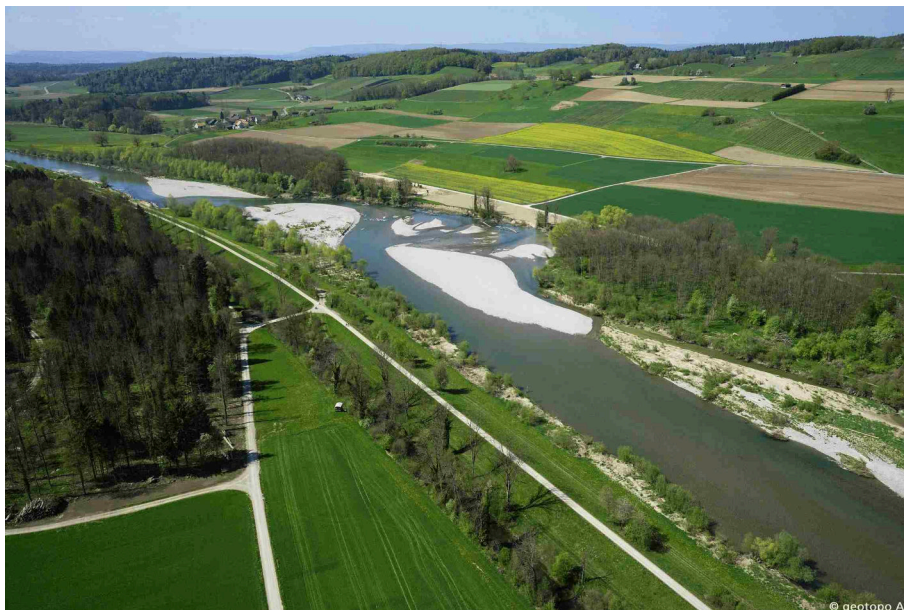
Figure 6.3 River widening at the River Thur near Altikon (ZH) in 2014, source: C. Herrmann, BHAtteam Ingenieure AG, Frauenfeld
