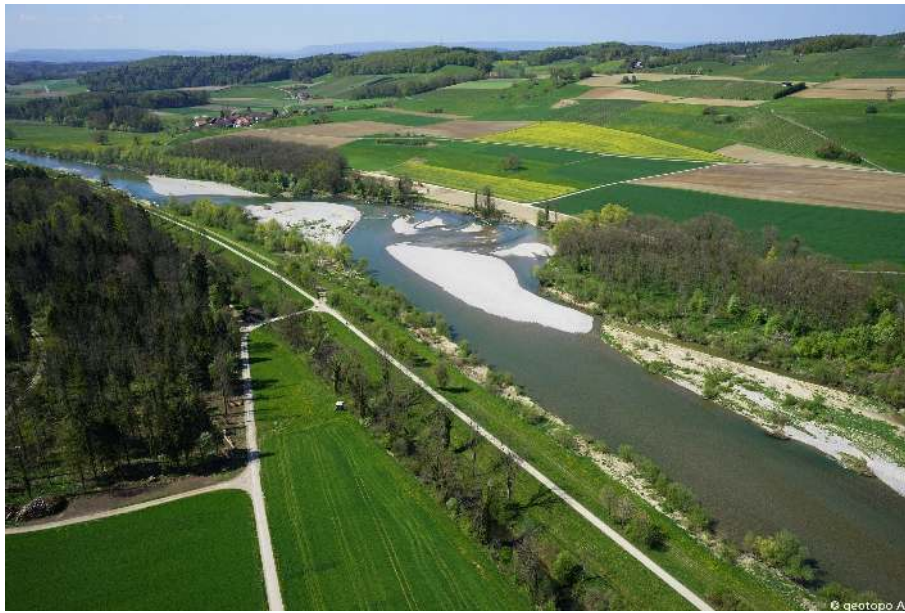
Figure 4.3 River widening at the River Thur near Altikon (ZH) in 2014, source: C. Herrmann, BHAteam Ingenieure AG, Frauenfeld
