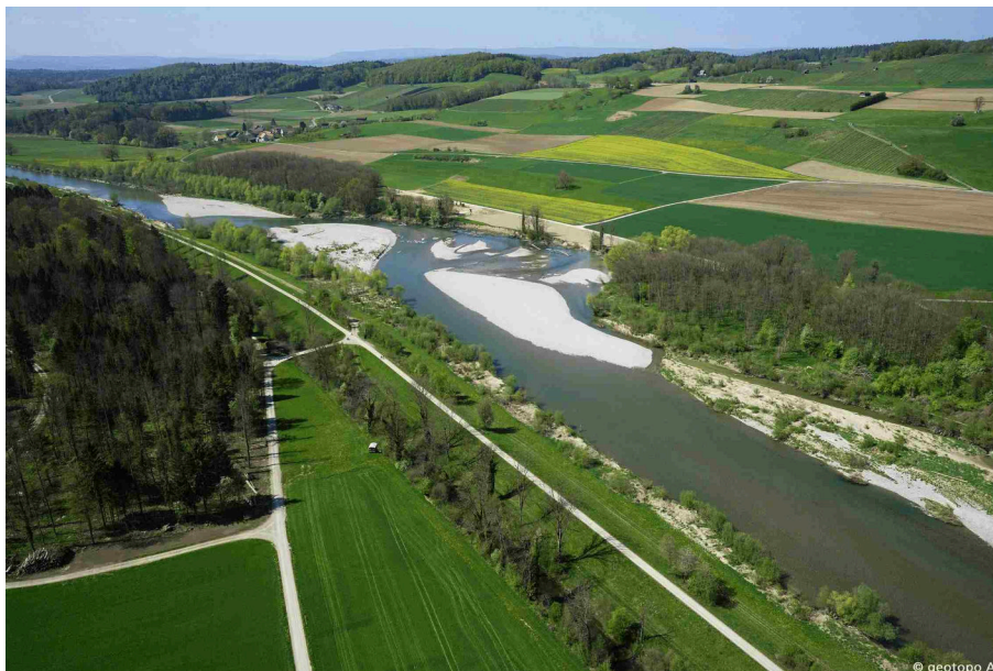
Figure 6.3 River widening at the River Thur near Altikon (ZH) in 2014, source: C. Herrmann, BHAteam Ingenieure AG, Frauenfeld
